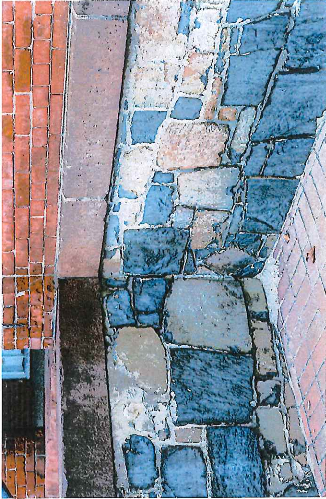
Front Steps/Foundation Repointing
