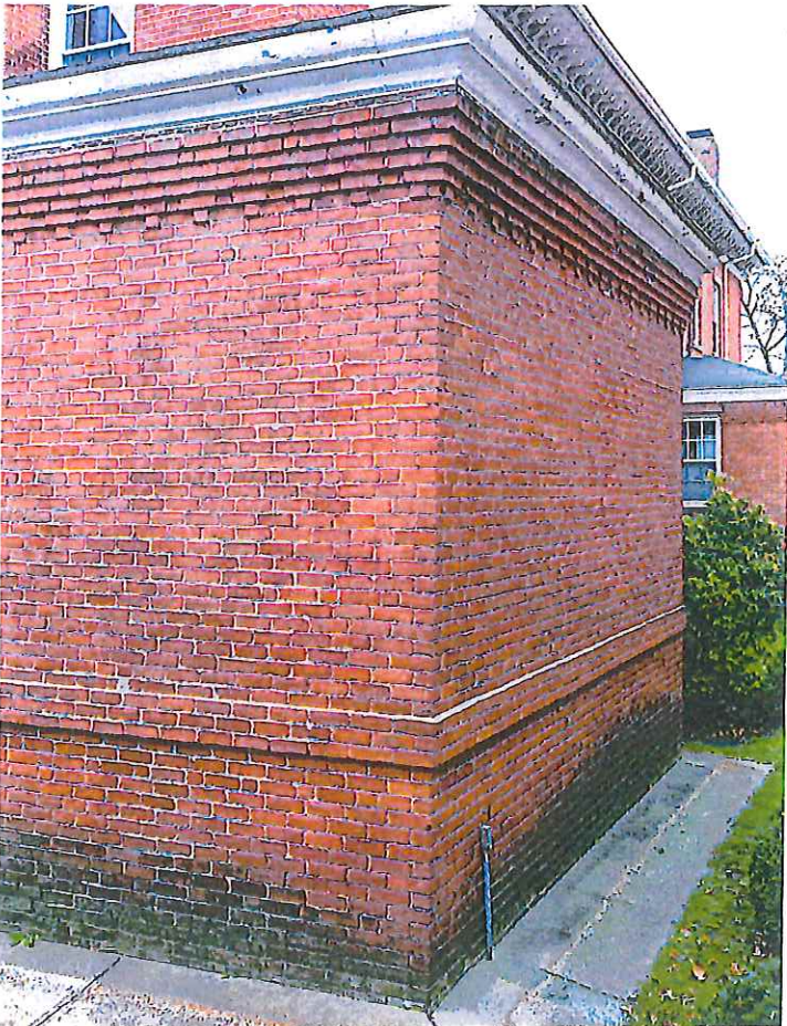
North Near Front - Re-set/Repoint Bricks
