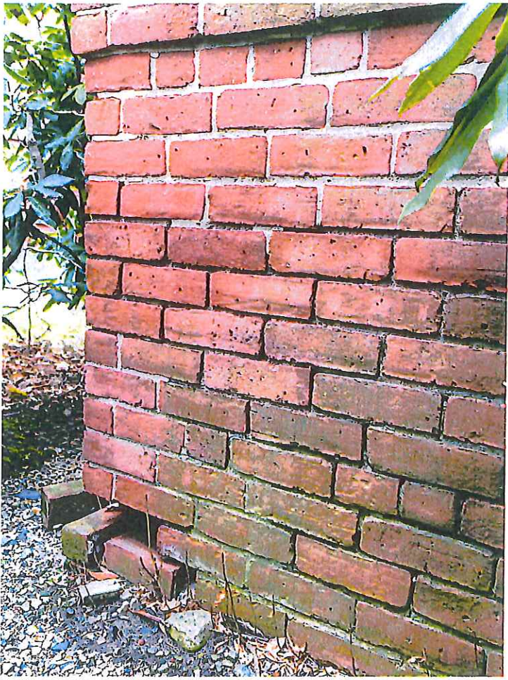
North Near Front - Re-set/Repoint Bricks
