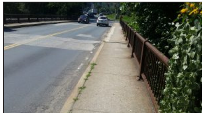
A portion of Cowles Bridge, which is along Southwick Road.
