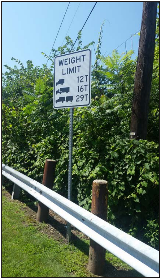
The posted weight limit on Cowles Bridge.
