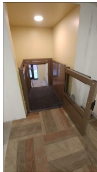
An elevator for improved handicap access at the Westfield Athenaeum.
