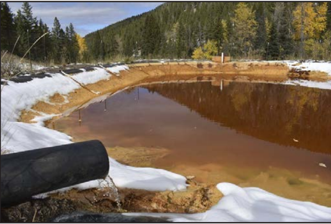
In this Oct. 12, 2018 photo, water contaminated with arsenic, lead and zinc flows from a pipe out of the Lee Mountain mine and into a holding pond near Rimini, Mont. The community is part of the Upper Tenmile Creek Superfund site, where dozens of abandoned mines have left water supplies polluted and residents must use bottled water. (AP Photo/Matthew Brown)
